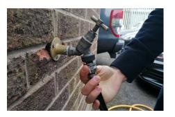
Connect the RED hose from the waste water outlet and direct to a drain or nearby soakaway
